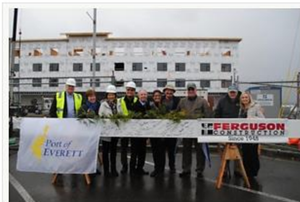
Port officials, hotel owners and architects and elected officials all signed the final beam before it was placed. Photo courtesy Port of Everett.
